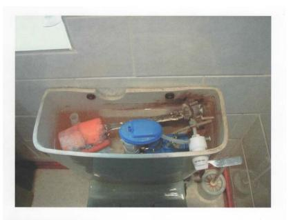
Plate 3.3: The Peter Brann Device The dial selector around the toilet handle determines the size of the flush, based upon the length of three tubes which extend below the device (not visible). The sipon is broken when water level in the cistern falls below the bottom of the tube selected.
